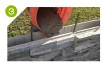
Fill cavities with concrete grout if desired height is more than three blocks tall
